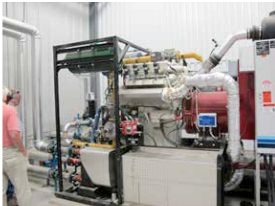
Engine designed to run on bio-gas, used to produce electricity
